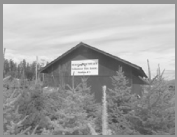
Hall Mountain Volunteer Fire Association Station #1
