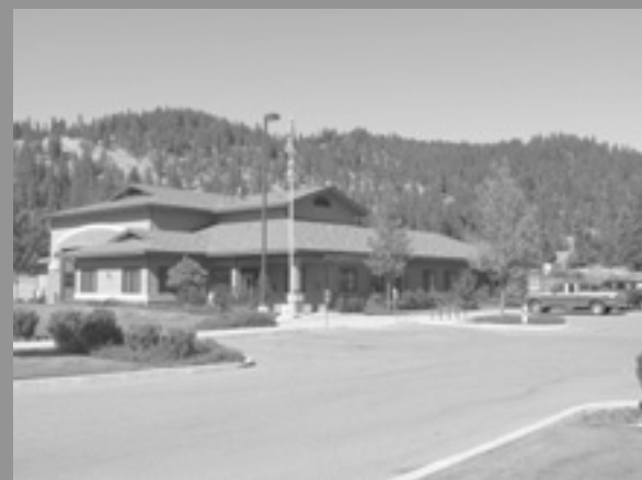
Coeur d'Alene Fire Department Station #3
