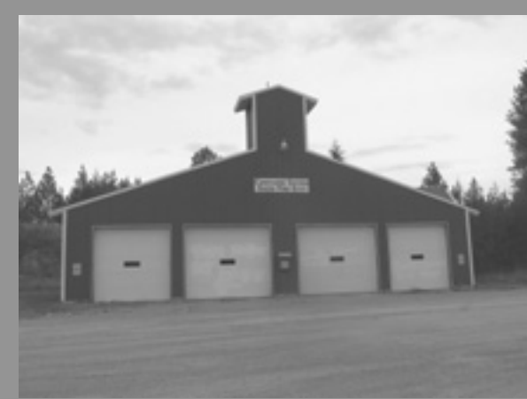
Sagle Fire District - Careywood Station
