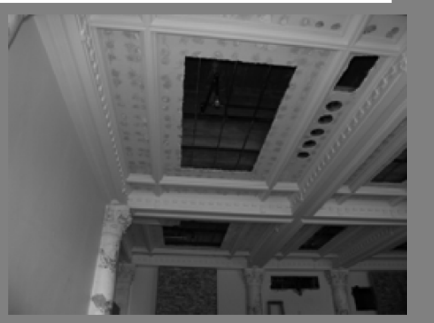
Capitol renovation includes addition of fire sprinkler system (AES).
