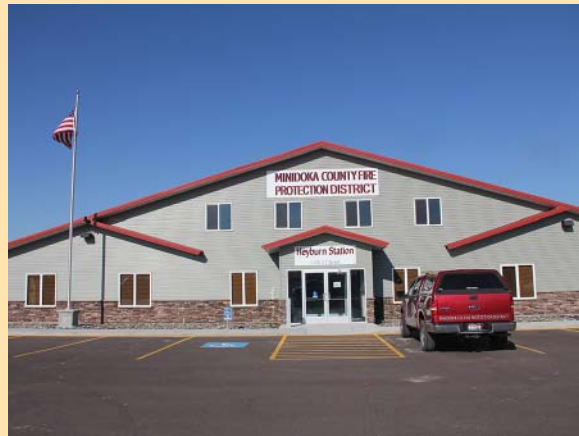
Minidoka County FPD - Heyburn Station
