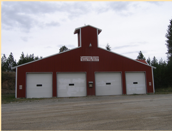
Sagle Fire District - Careywood Station
