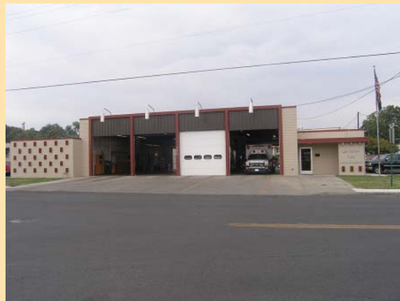
Lewiston Fire Department - Station #1
