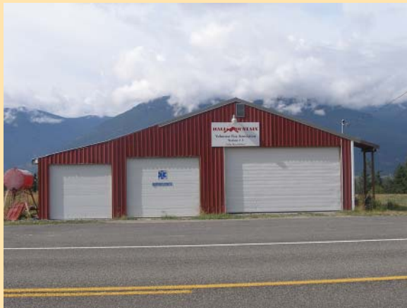
Hall Mountain Volunteer Fire Association Station #2
