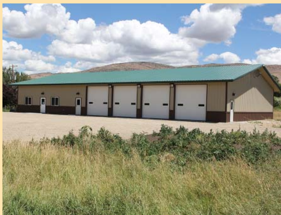
Gem County Fire Protection District #2 Sweet-Montour Station
