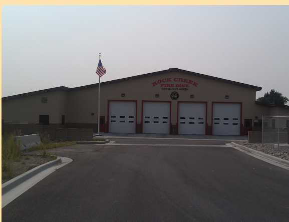
Rock Creek Rural Fire Department - Station #1
