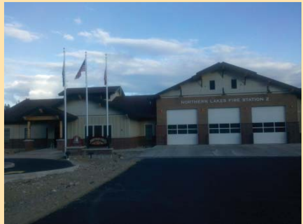
Northern Lakes Fire District - Station #2
