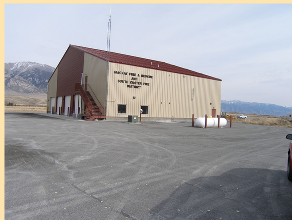
Mackay Fire and South Custer Fire
