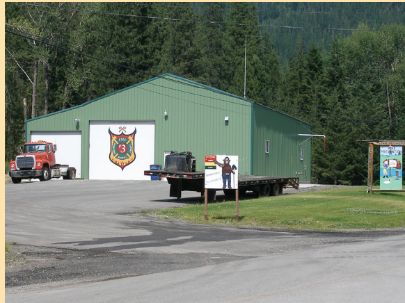
Shoshone County Fire Protection District Station #3 - Mullan
