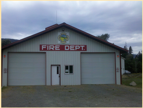
South Boundary Fire Protection District - Deep Creek Rd
