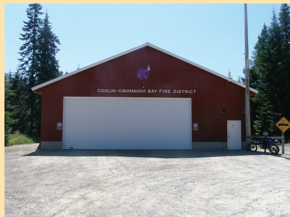
Coolin-Cavanaugh Bay Fire Protection District
