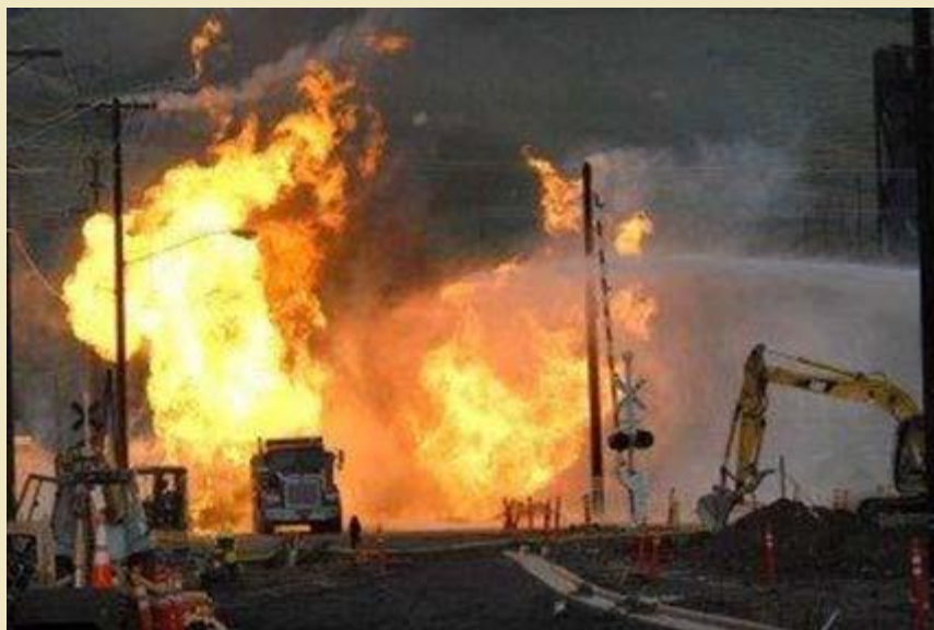
Gas Line Fire - Nez Perce County Photo provided by Lewiston Fire Department
