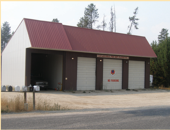
Cascade Rural Fire Protection District Station #2
