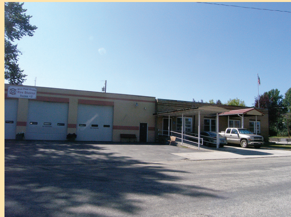
West Pend Oreille Fire District Station #2
