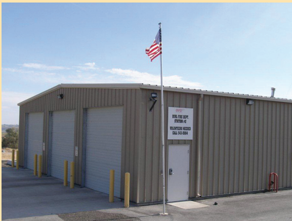
Buhl Fire Department - Station #2
