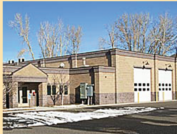
Wood River Fire & Rescue - Station #3
