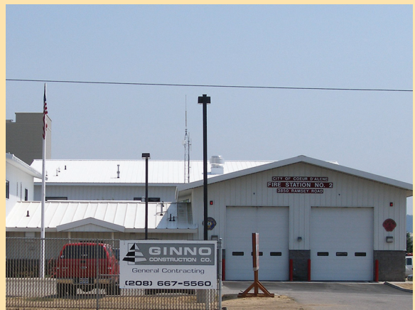
Coeur d'Alene Fire Department Station #2 - Ramsey Road
