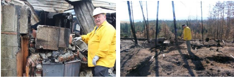
Left: Deputy Bill Steele examines a chimney and flue for indicators that it may be connected to the cause of this fire.
